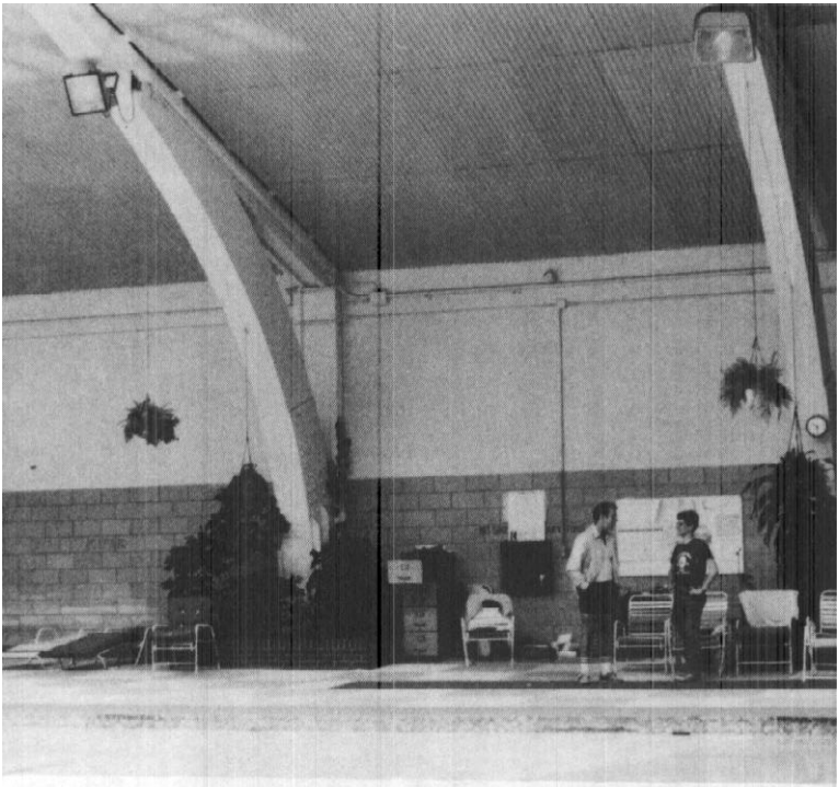
Figure 4-2. Glulam arches with rating 100. No sign of deflection or deterioration.
