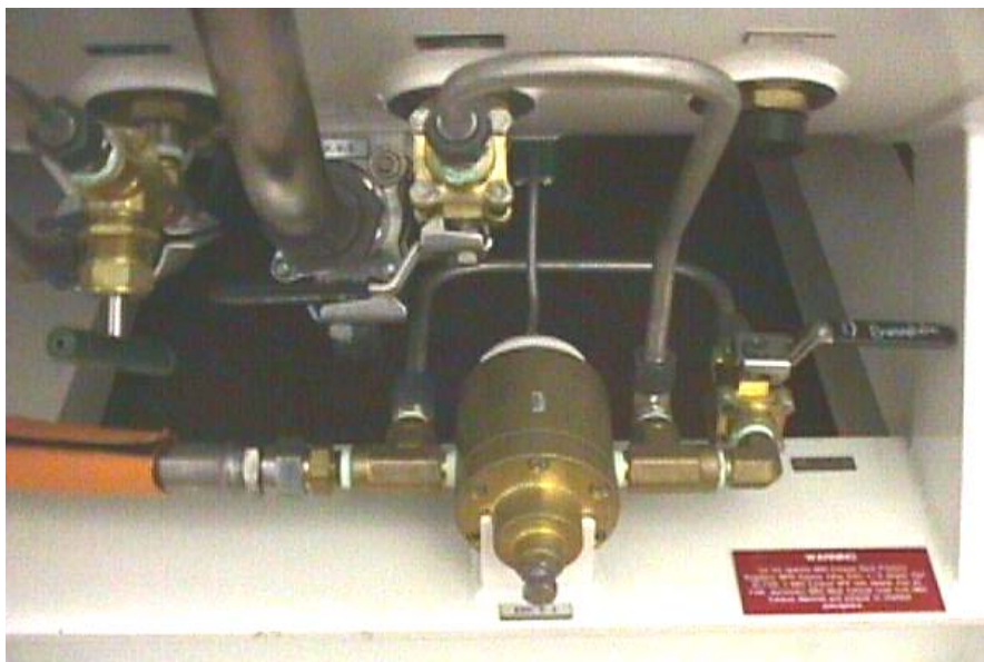
Figure 3-20. BIBS Exhaust Back Pressure Regulator
