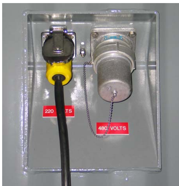
Figure 2-2. Power Receptacle Box
