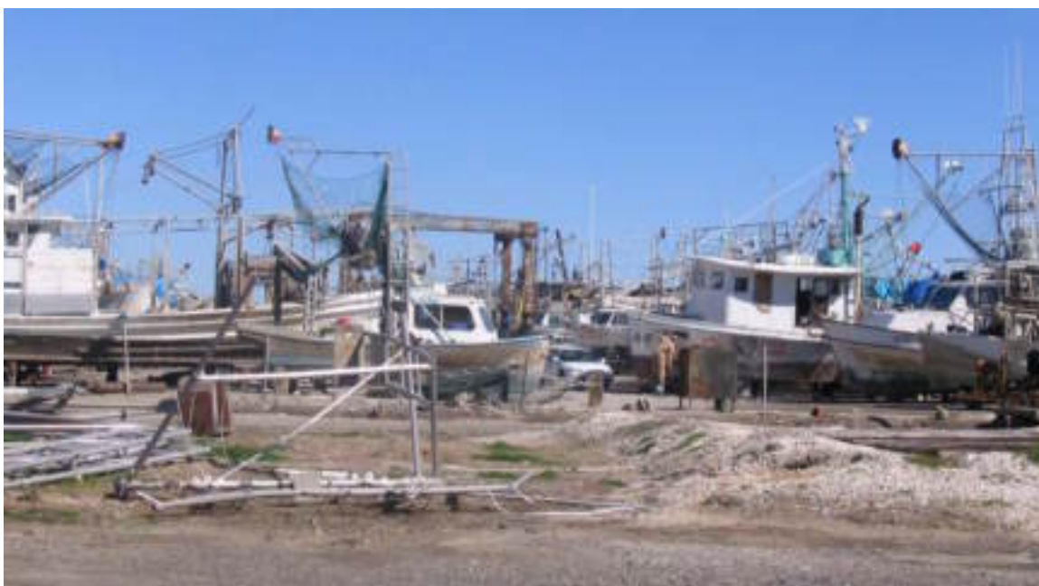
Figure 5-13. Recovered boats blocked and stored in the boatyard in Empire, LA.
