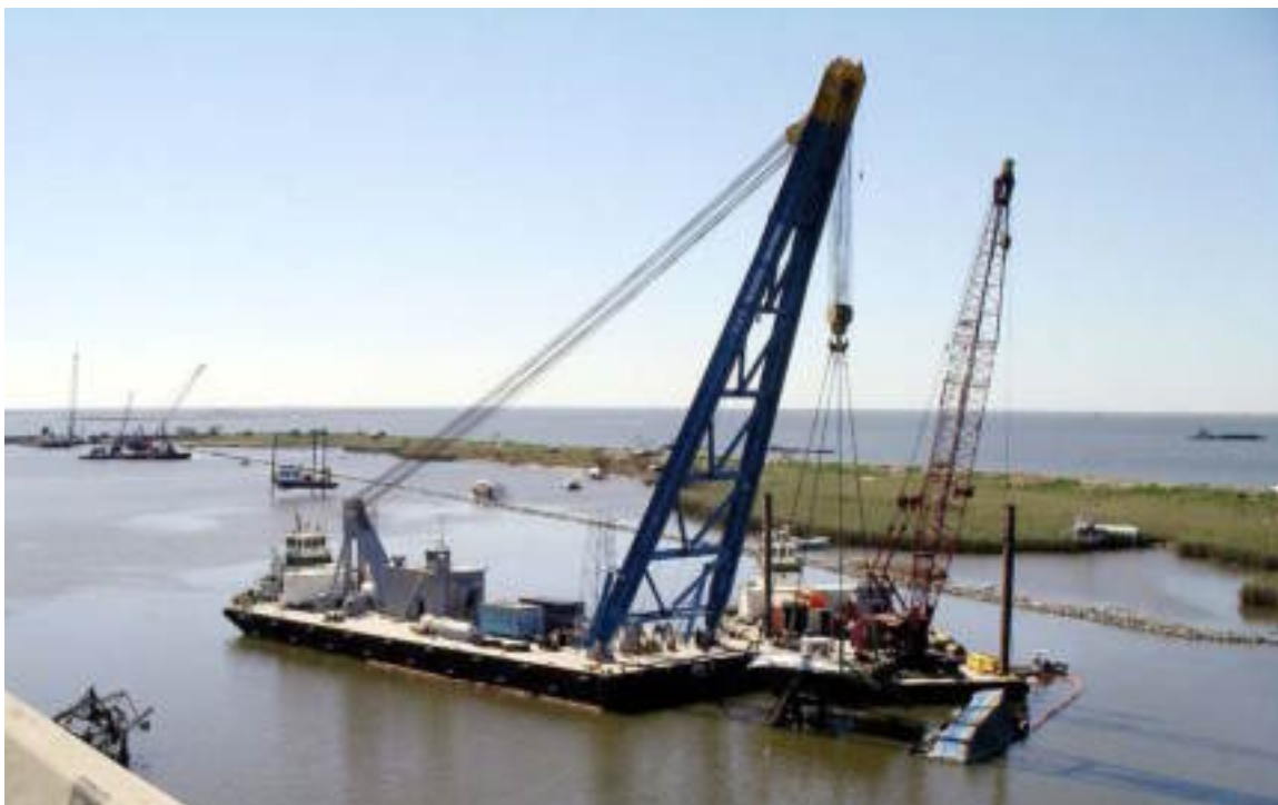
Figure 5-12. T&T's Big and George T working on a lift on the westward approach to Empire, LA.
