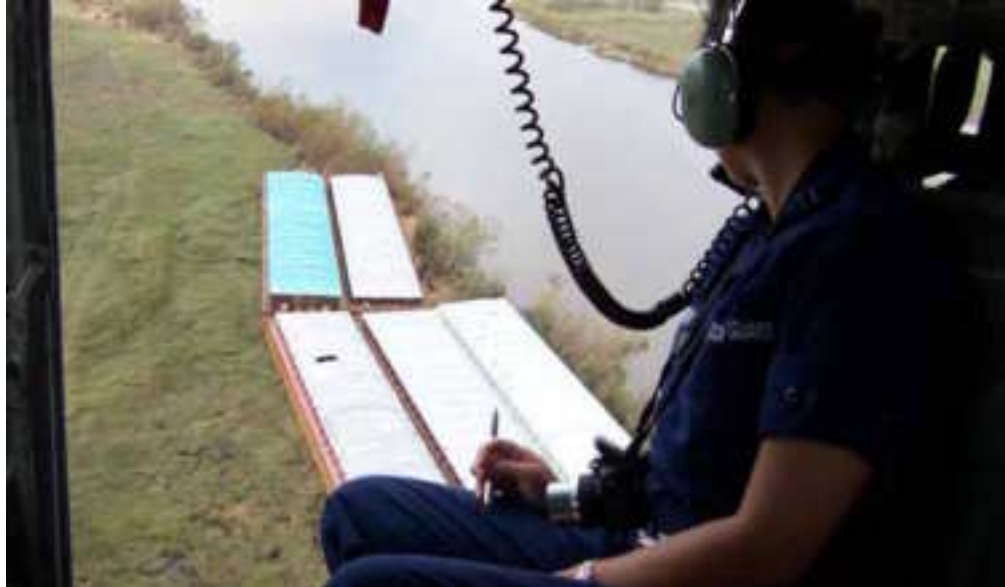
Figure 4-7. Hurricane Rita damage as viewed from the Bell 212 chartered helicopter.
