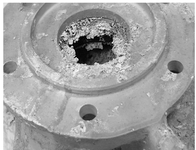
Figure 3-24. Magnesium Corrosion Products
