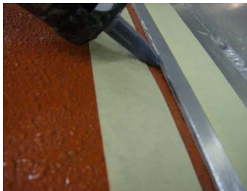
Figures 2 & 3: Current configuration of RB-S Collar/Fin interface, showing installation and details of Adhesive seal between the collar and Lower Flange.
