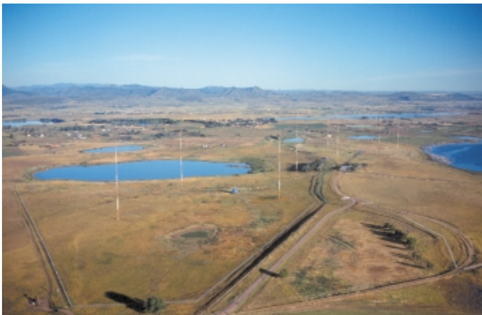
Figure 2.1. Aerial View of WWVB/WWV Station Site
