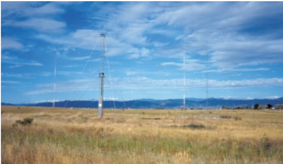
Figure 3.4. 15 MHz WWV Antenna (WWVB Towers in Background)
