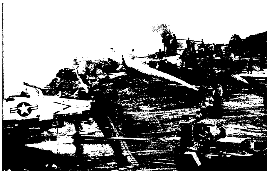
Figure 3. Aftermath of U.S.S. Forrestal EMI incident.
