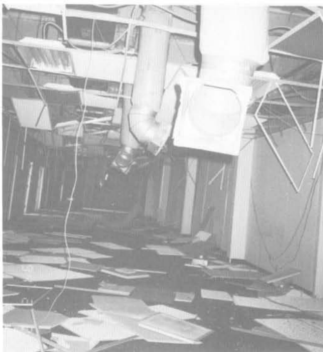
Air diffusers fell to the floor. Earthquake Damage: 1994, Northridge, California Photo Credit: Wiss, Janney, Elstner Associates, Inc
