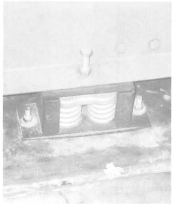
Chiller mount with no uplift resistance and insufficient or no shear resistance. Photo Credit: Wiss, Janney, Elstner Associates, Inc.
