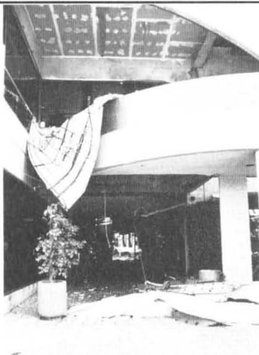
Failure of suspended ceiling and light fixtures in furniture store Earthquake Damage: 1994, Northridge, California Photo Credit: William McKeivitt
