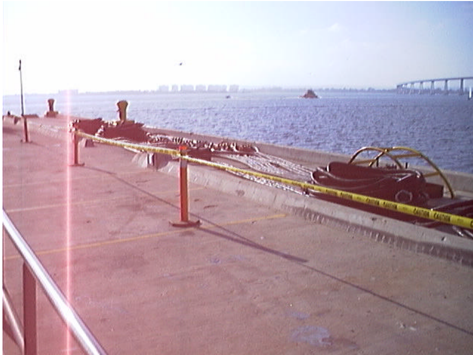
Picture L. Cable protection safety barricades.
