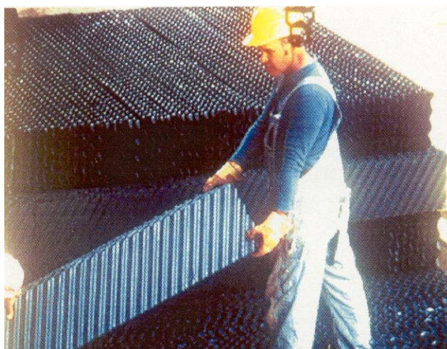
Figure 4-11. High-Efficiency Cooling Tower Film Fill
