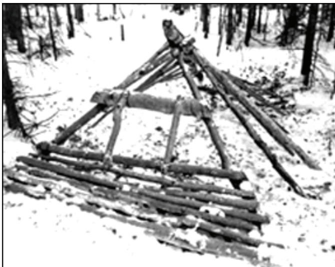
Figure 2-1. Frame of infrared counterdetection (thermal) shelter
